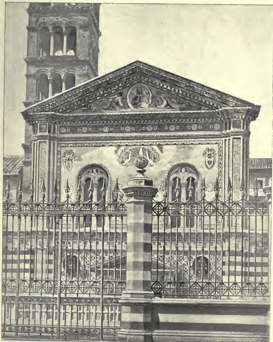
CHURCH OF STA. PUDENTIANA, ROME. Showing facade in mosaic.
