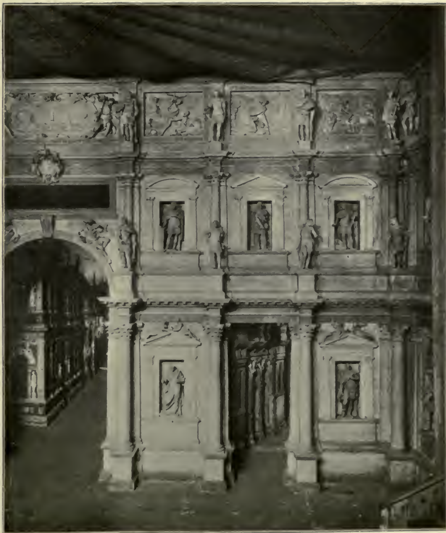
FIG. 16.—PORTION OF THE STAGE SETTING, TEATRO OLIMPICO, VICENZA. Showing Palladio's use of the entasis in all columns and pilasters. Compare Fig. 15.
