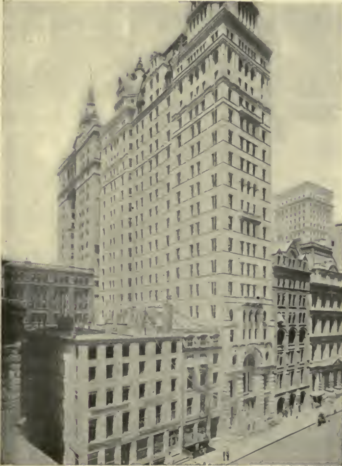
THE COMMERCIAL CABLE BUILDING. Broad Street, New York City.
