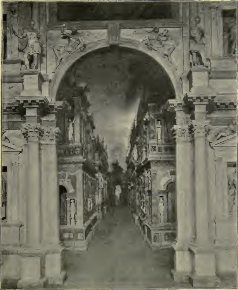
FIG. 15.—PORTION OF THE STAGE SETTING, TEATRO OLIMPICO, VICENZA. Showing a horse-shoe bend in the profile of arch and pier, as result of Palladio's use of the entasis in pilasters. Compare Fig. 16.
