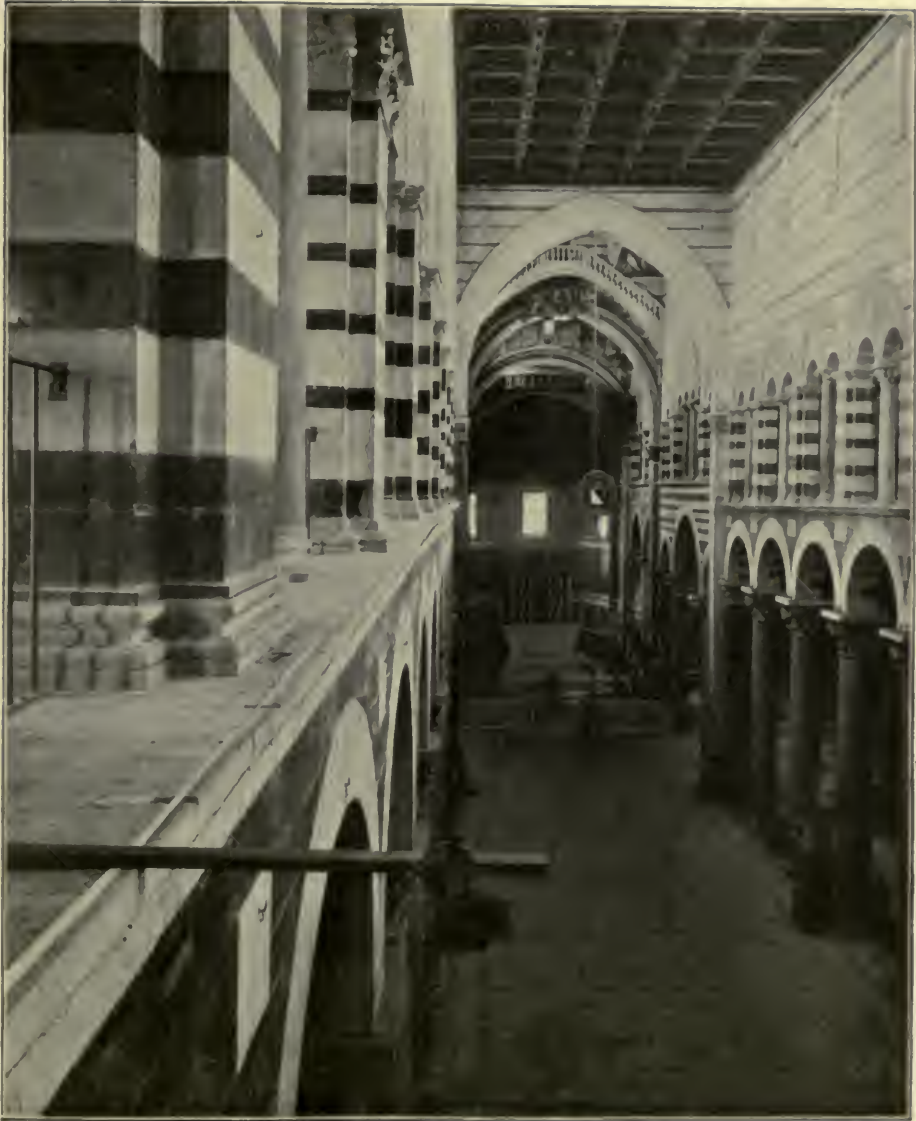
FIG. 7.—NAVE OF THE PISA CATHEDRAL AND THE NORTH GALLERY. Showing the entasis in the profiles of the pilasters at the transept (also showing the bend in elevation of the north gallery).
