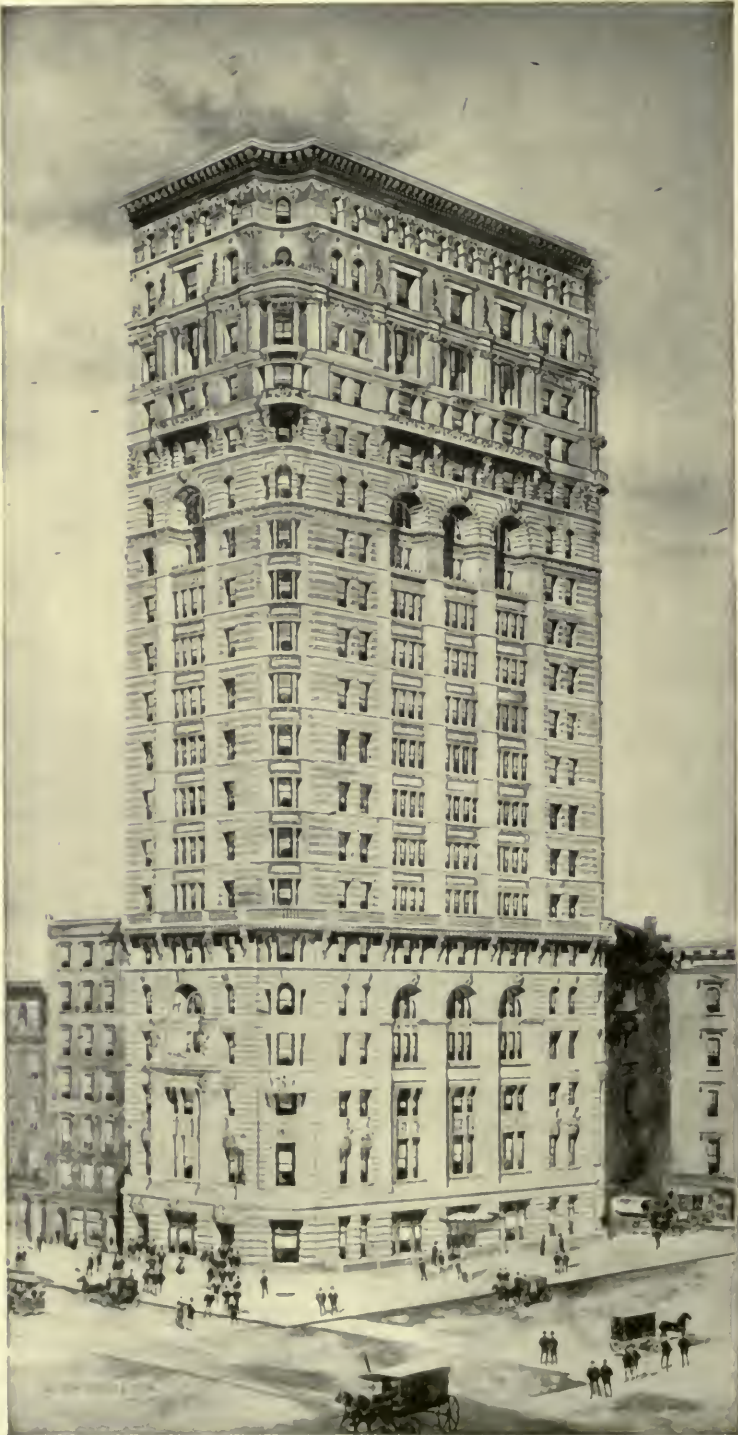
THE DUN BUILDING. Now erecting N. E. corner Broadway and Reade St.
