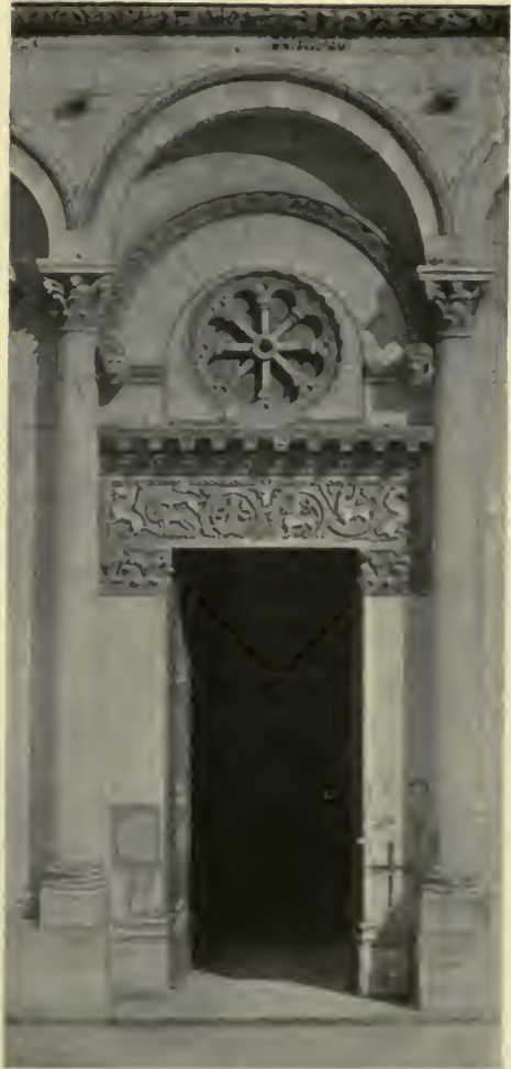
FIG. 3.—DETAIL OF FACADE, S. MICHELE, LUCCA: The engaged mediæval columns have an entasis.
