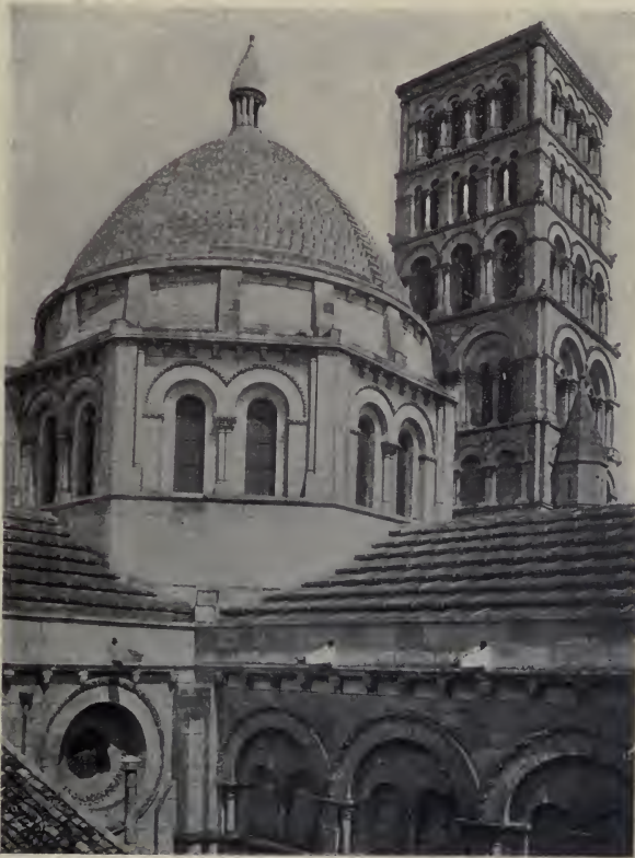
ANGOULÊME CATHEDRAL.—VIEW OF DOME AND TOWER.
