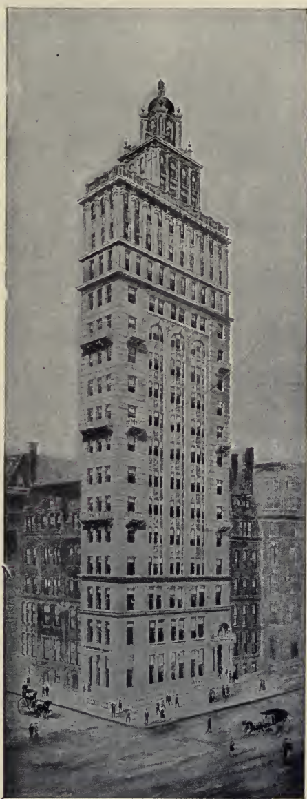
149. The Gillender Building. Berg & Clark, Architects. A tall office building subdivided into five parts.
