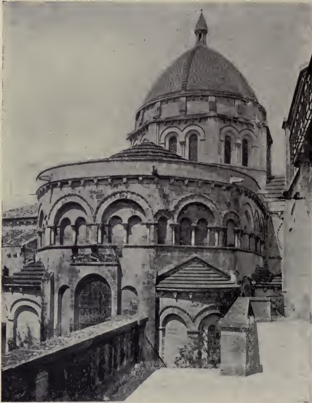
ANGOULÊME CATHEDRAL.—VIEW OF APSE AND DOME, NORTH SIDE.
