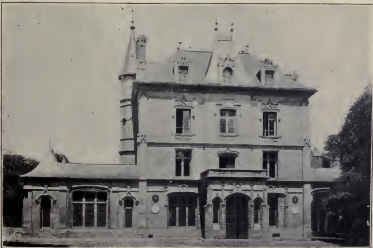
90. Mass, with a single appendage. The one-story portion on the left side is the appendage.
