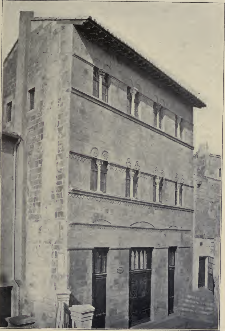
136. Romanesque House, St. Gilles, France. Showing the unifying effect of a single large cornice.
