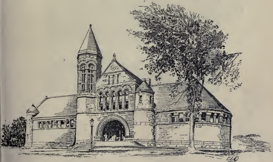
62. Billing's Library, Burlington, Vt. H. H. Richardson, Architect. The gable is the principal mass in this composition. The taller tower is a single subordinate mass placed unsymmetrically. It is to be regarded as single because the smaller and rather anomalous tower is not large enough to constitute with the other a group of two.
