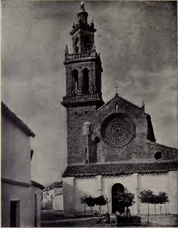
63. A single tower placed unsymmetrically.
