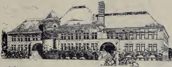
94. Pillsbury Science Hall, Minneapolis. L. S. Buffington, Architect. The high central part is the main mass. The tower is an unsymmetrical subordinate mass. The wings are two appendages.
