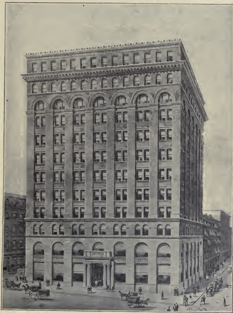
148. The Woodbridge Building. Clinton & Russell, Architects, William Street, New York City. A five-part subdivision.
