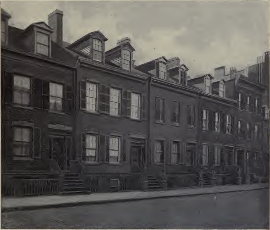
NOS. 16 TO 20 VANDAM STREET.
