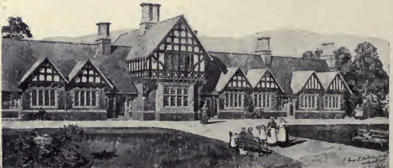
279. Llewellyn Almshouses. Double gabled treatment united by heavy overhang of gables.
