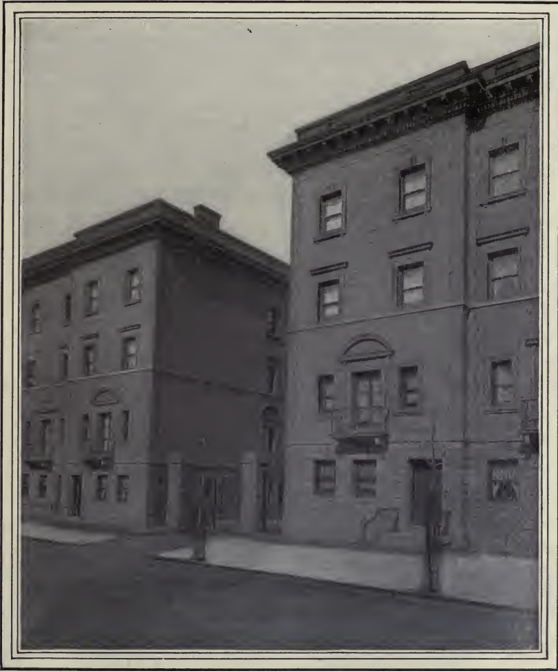
NOS. 217 AND 219 WEST 139TH STREET.
