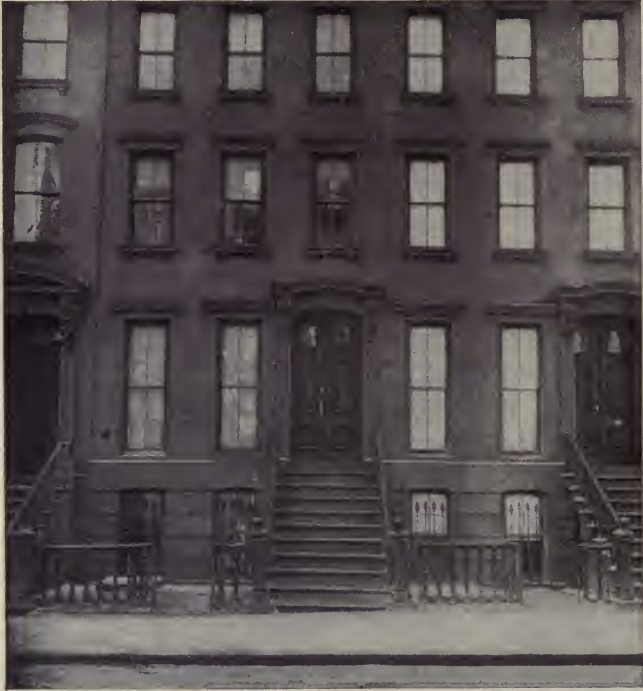
NO. 238 EAST 51ST STREET.
