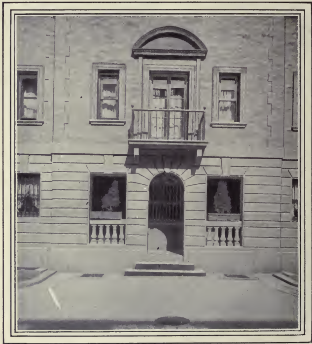
NO. 233 WEST 139TH STREET.
